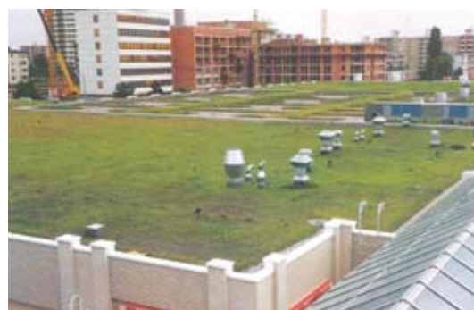
2 Shopping centre (Germany)
